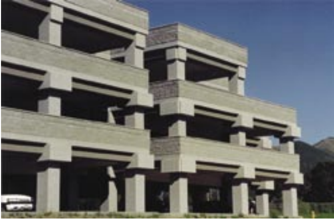
Fig. 6: Ground-level view of completed structure
