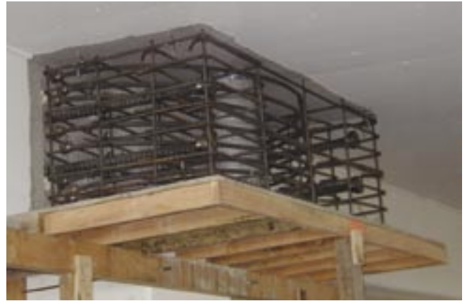
Fig. 7: Reinforcing and soffit form at interior column
