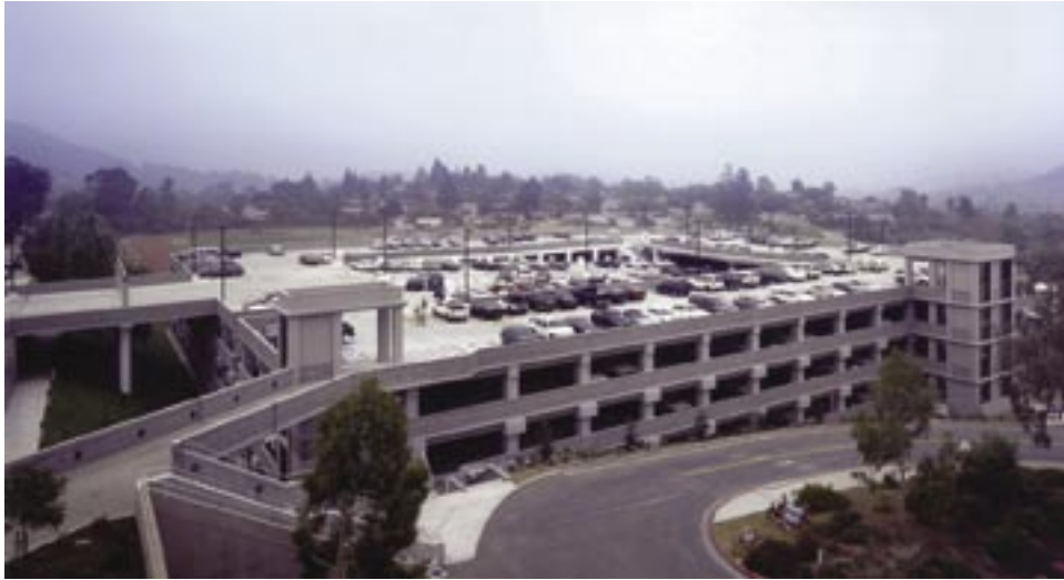
Fig. 2: View of the completed parking structure with reinforced joints at the lower two levels
